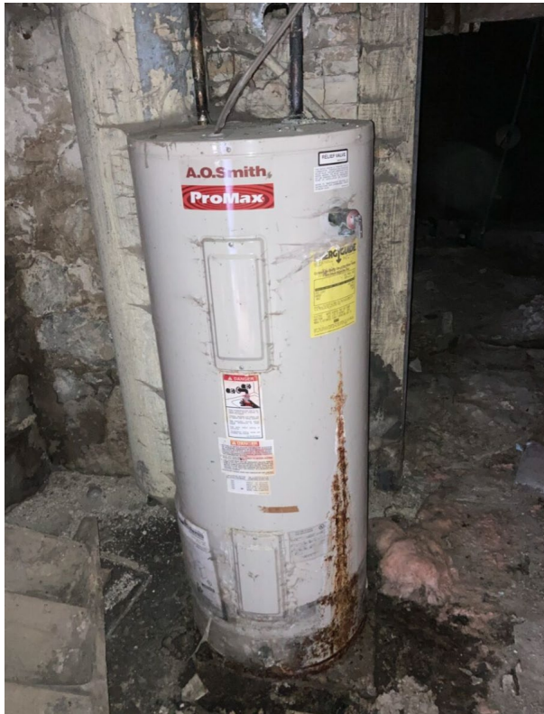
Water Heater Before
